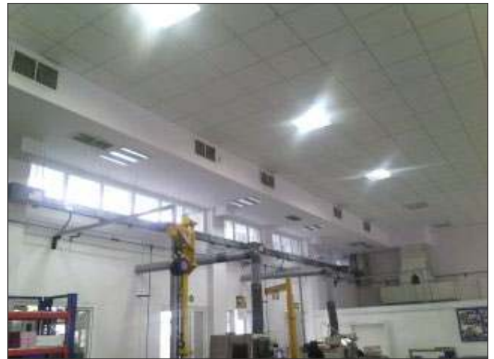
Ducting layout inside the carbide grinding floor
