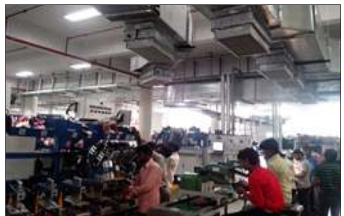
Ducting layout inside the factory
