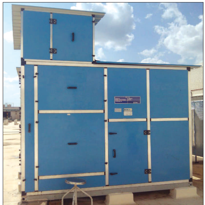
15,000 CFM HMX-Ambiator installed at Himalaya's Bangalore plant
