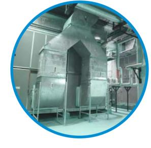
Reduces fresh air load on AHU coils resulting in reduction in energy consumption
