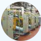
Air compressors/ DG rooms
