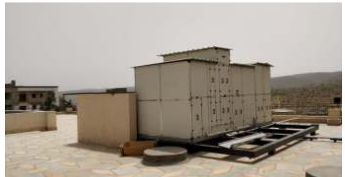
Machine installed at AAETI
